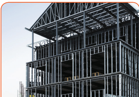
Buildings with steel frames are generally considered more resistant to earthquakes
