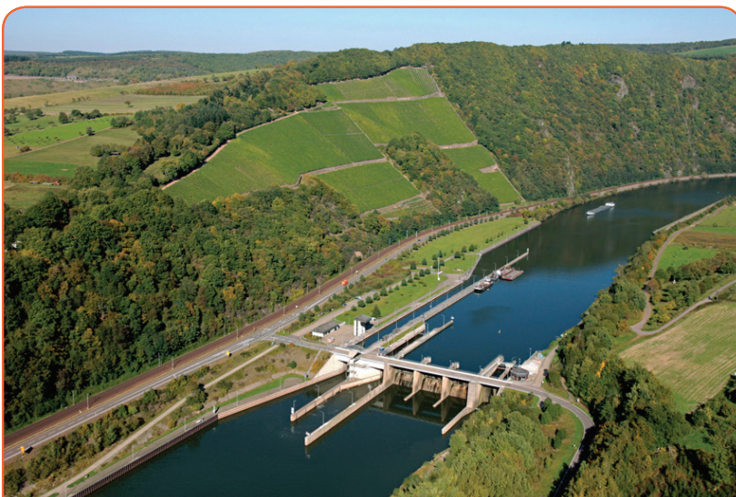
Dams situated on rivers trap water and then release it under pressure, passing it through turbines which are connected to generators
