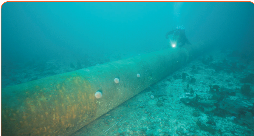
Pipelines can transport carbon dioxide in three states: gaseous, liquid and solid
