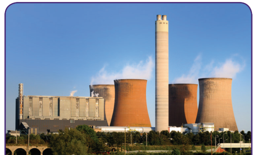
A power station and its cooling towers
