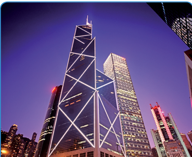
Triangles are an integral part of the design and construction of the Bank of China.
